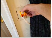
(2) The garage interior outlets were grounded but were not GFCI protected. Recommend updating garage outlets to have GFCI protection.
