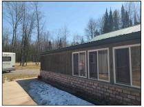
(2) Downspout extensions are needed to move water away from the foundation.
