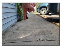
(3) There were a few areas around the house where the grading was low. Recommend correcting the grading around the home for proper drainage away from the foundation.
