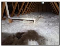
(2) The attic access was not very well insulated, and was not sealed adequately. Recommend installing a properly insulated and air-tight access for heating cost efficiency and to help prevent the escape of warm and/or moist air into the attic.
