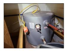
(2) Temperature-Pressure relief valve extension pipe is missing on water heater, extension pipe should be 4"- 6" off the floor. Install extension pipe as needed.
