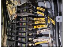
(2) A 30 amp breaker in the electrical panel was oversized for the connected 12 gauge wires. The breaker was for the whirlpool tub. This may be allowed based on the recommendation of the whirlpool manufacturers recommendations. A licensed electrician should further evaluate and repair as or if needed.
