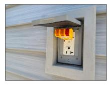
(2) The exterior outlet at the rear entrance was not GFCI protected. Recommend updating exterior outlets to GFCIs.
