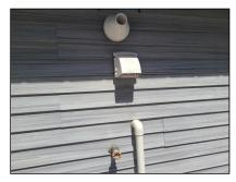
(2) Bathroom exhaust fans were vented to the exterior of house.
