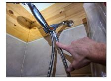
(4) The diverter valve in the shower was leaking. The inside components of these mechanisms can often be replaced.
