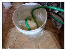
(2) A back pressure test was performed by shutting the water off to the house for approximately five minutes to test the pressure between the pressure tank and the well. The back pressure test was satisfactory.
